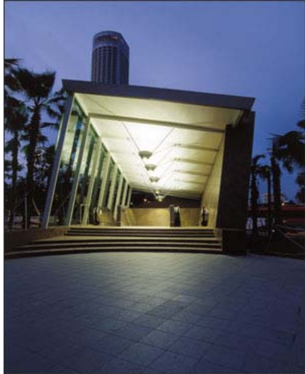
Pedestrian underpasses at The Esplanade were completed by Tew Kim Thai Construction.
