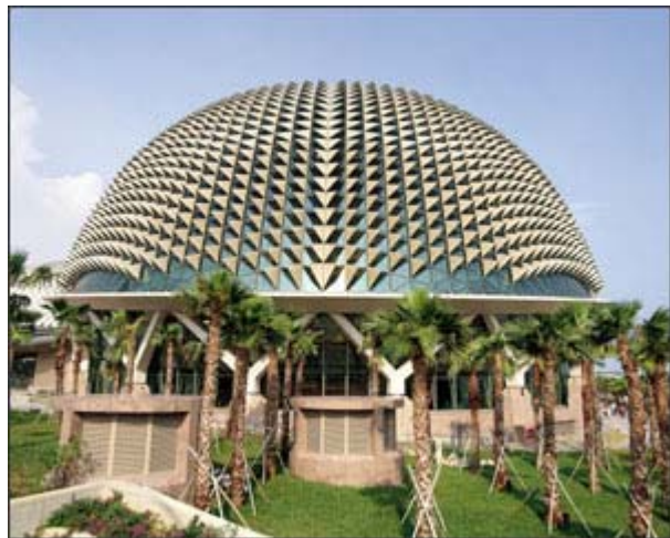
Mero Asia Pacific says the shading envelope was designed to ensure it would fulfil light and thermal transfer requirements, as well as aesthetic aspects, with the gradual opening, closing, rising and falling of the shading elements.
