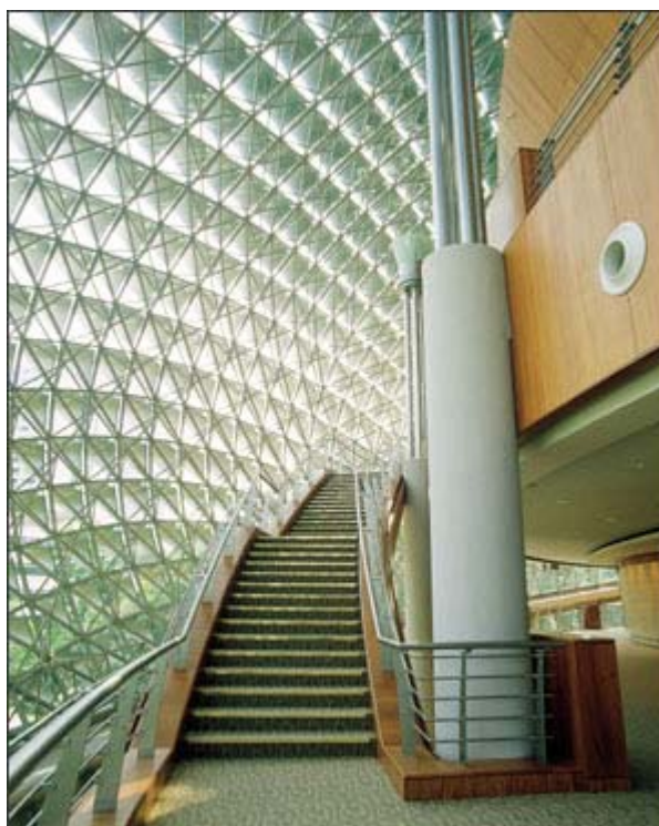
Each dome is a double-layered space frame featuring a triangular grid of rhombi. The Mero spherical node and circular tubes system connects the internal and external layers.
