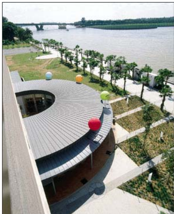
BHP Steel also supplied and installed the top roof of the J-shaped food court. Other roofing manufactured and installed by BHP Steel includes Colorbond Kliplok roofing.
