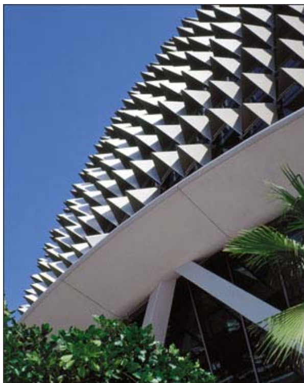
Aluminium pyramids provide a shading envelope for the interior of the complex.
