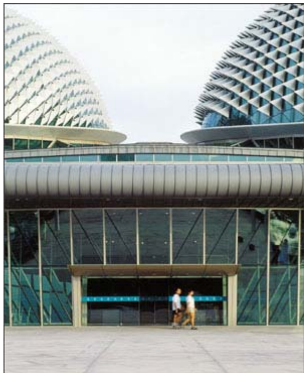
BHP Steel supplied and installed zinc titanium roofing for the public concourse. This standing seam roofing can be roll-formed as shown.
