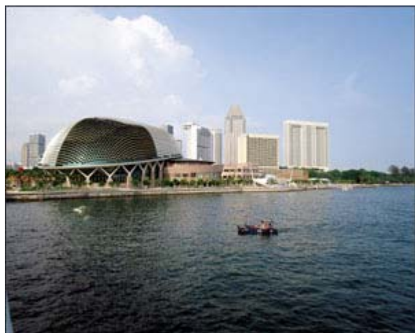
With its multi-faceted dome structure, The Esplanade - Theatres on the Bay makes a bold architectural statement. The steel, glass and aluminium structures were fabricated by Mero Asia Pacific.
