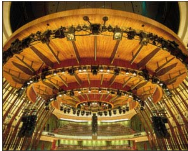
The spectacular Concert Hall canopy at The Esplanade features special effects finishes by Naa'im Holdings, the company responsible for much of the fitout.
